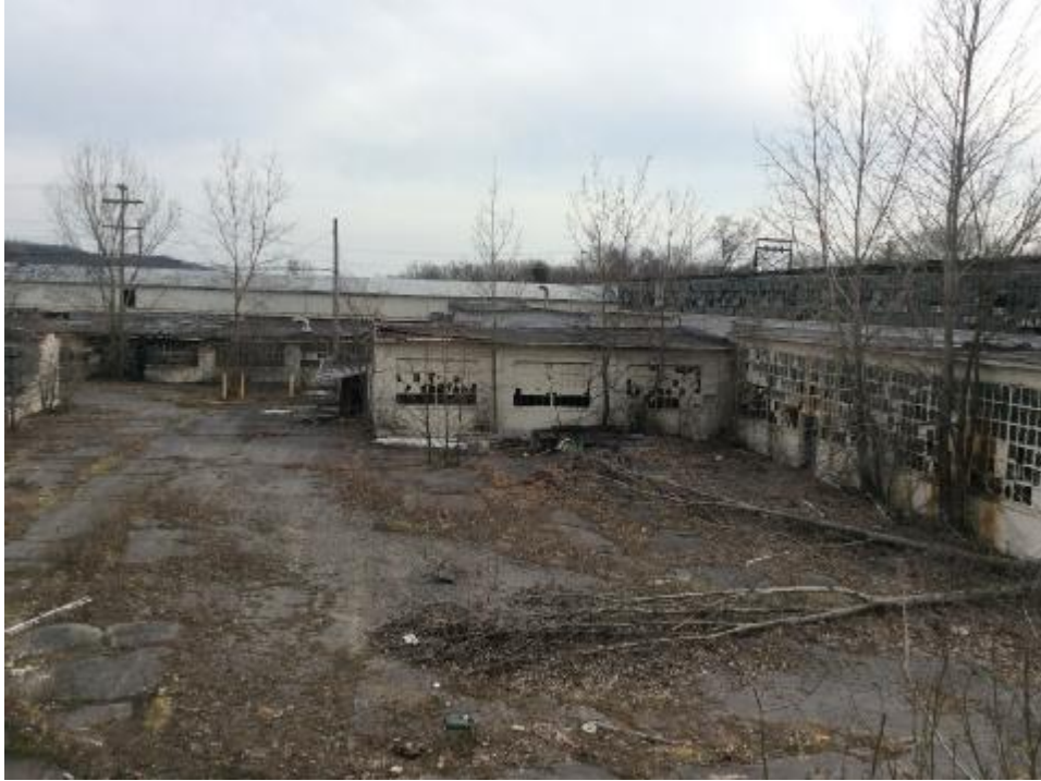
North elevation of main building
