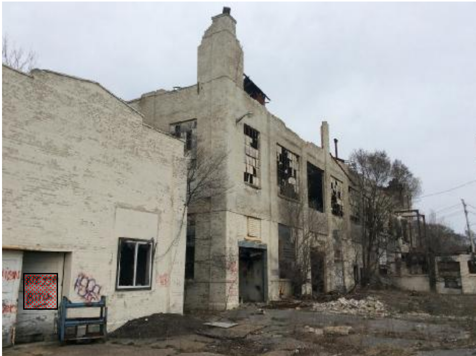
Scale house and Glendale Building looking northeast
