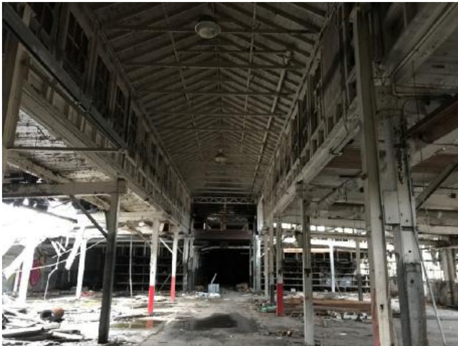
Interior view future office and training facility
