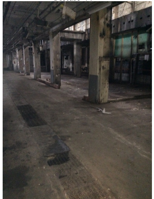
Example of typical floor drains.
