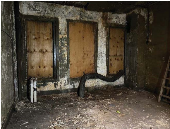
Image of the southern-facing boarded windows on the second floor
