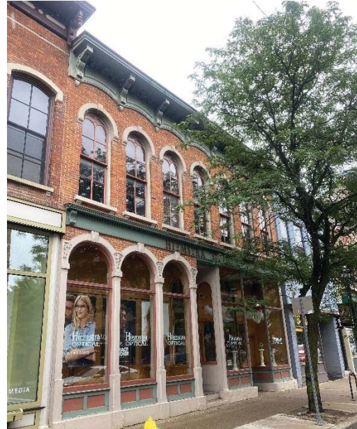
Image of the north-facing façade of the property
