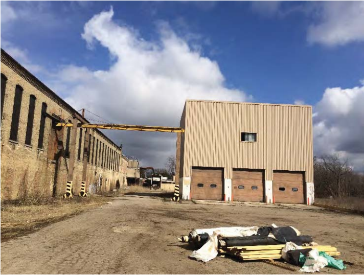
View north along the east side of the building to the sludge handling building.
