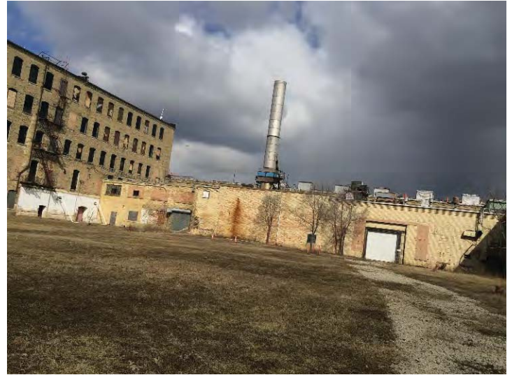
View north to the central area between the two wings. Machine, boiler and engine rooms in this area..
