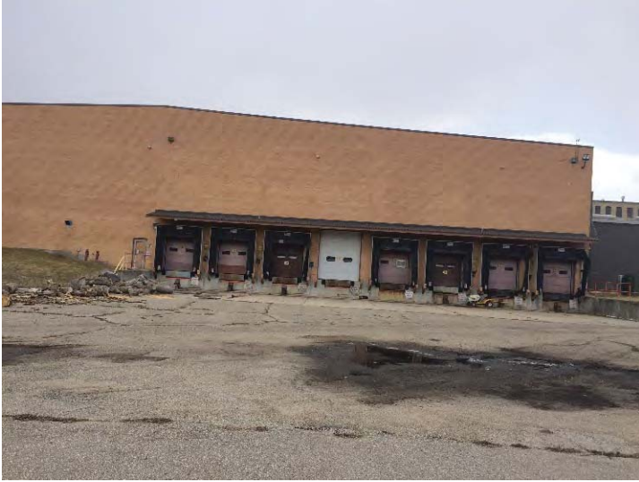
View east to the west side of the mill.
