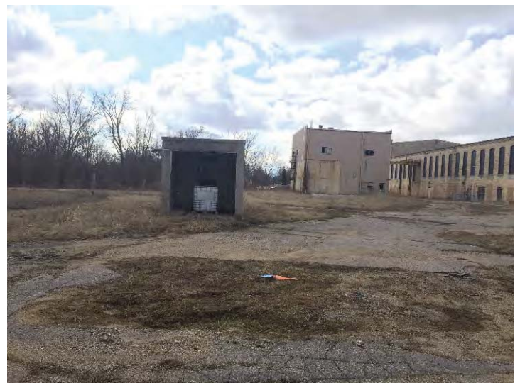
View south from the wastewater process building to the sludge handling building along the east side of the mill.
