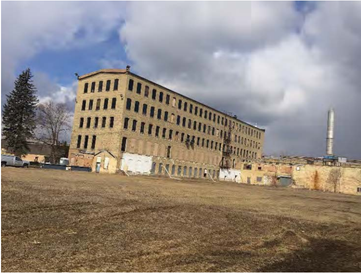
View northwest to the west wing of the mill.
