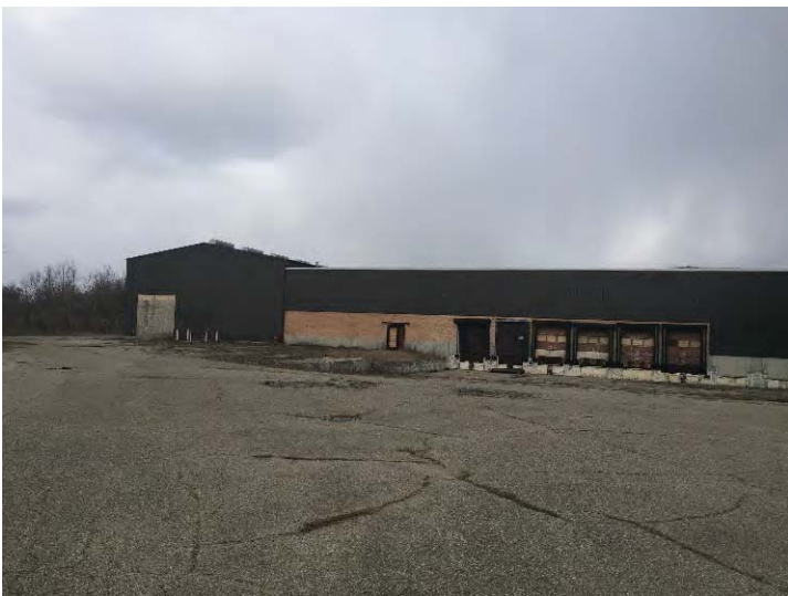
View north to the west end of the south side of the mill building.
