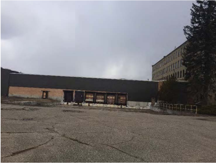
View north to the newer warehouse portion of the mill on the west side of the Property.
