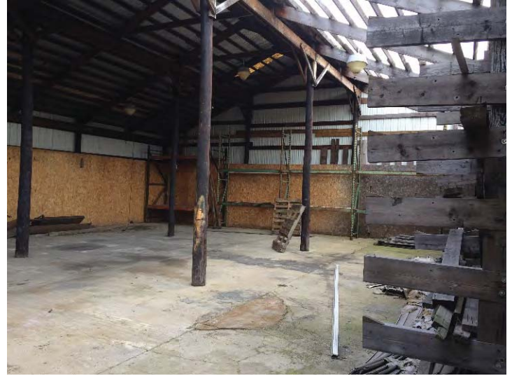
Interior of maintenance garage.
