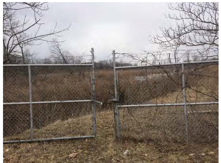
View west from the western edge of the Property to the adjoining former Emergency Overflow Area (EOA).
