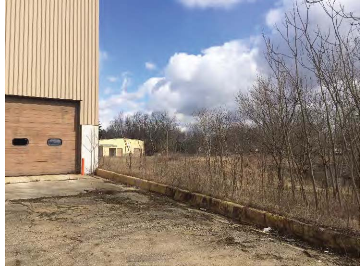
View north east of the sludge handling building with wastewater process building in the background.
