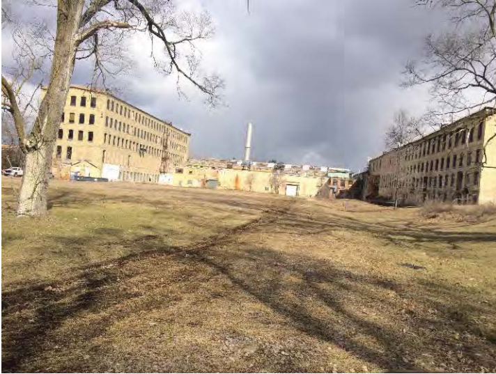
View north from entrance at West Highway Street.
