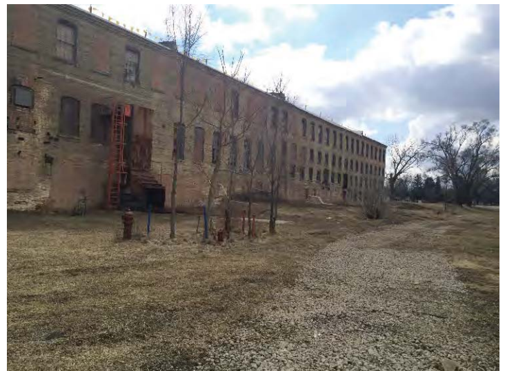
View southeast to the west side of the east wing.
