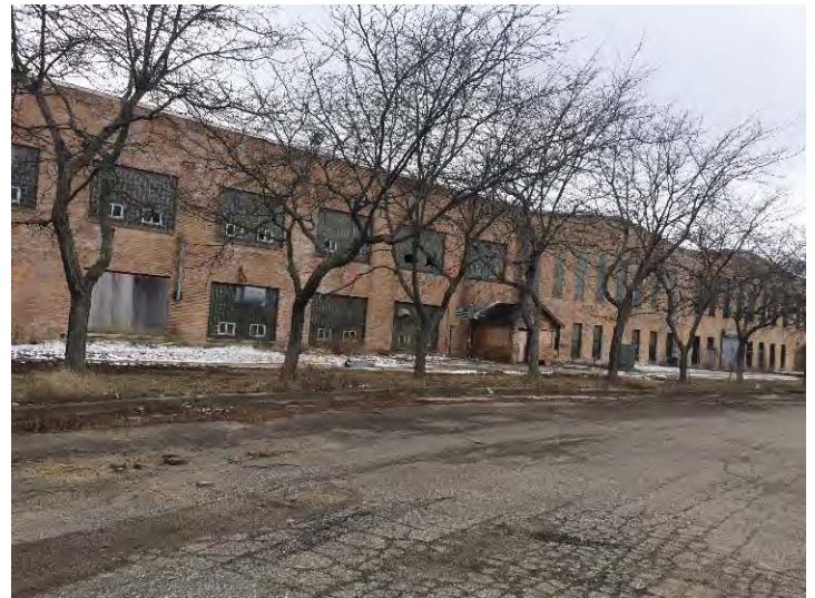
View southwest to the mill building, east portion.
