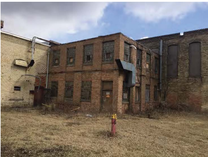
View northeast to the northeast corner of the "U" formed by the two wings. A cistern is located in this area.
