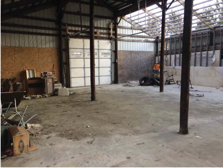
Interior of maintenance garage.
