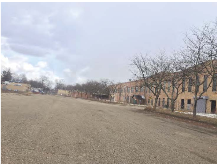
View east along the north side of the mill.
