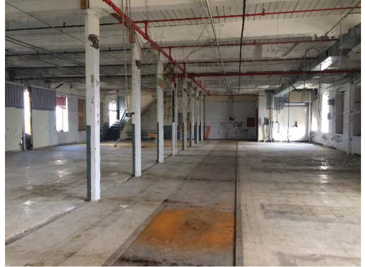
Typical interior of the sections in the east and west wings.
