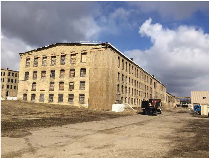
View north to east wing – oldest building section.
