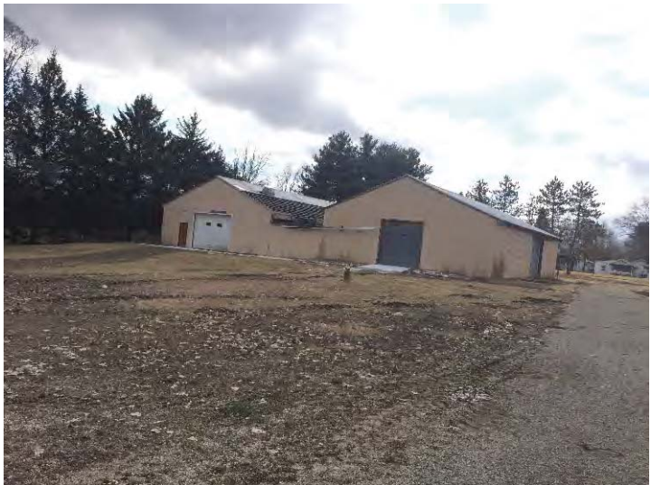
View south to the maintenance/storage building.
