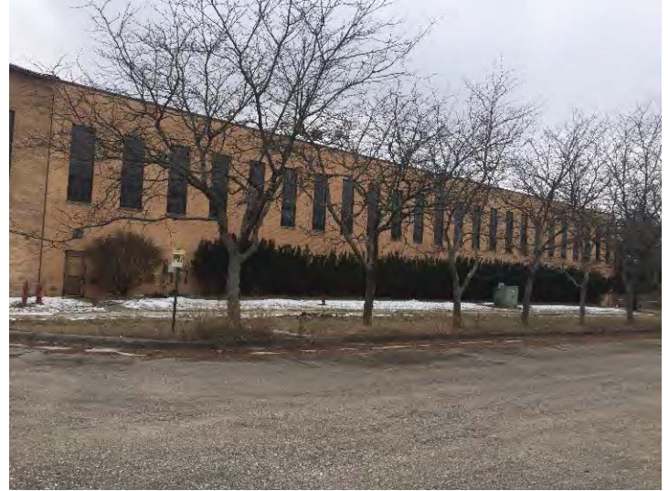
View southwest to the mill building, west half.
