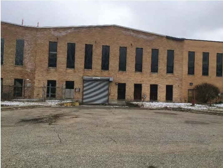
View south to the center of the mill building.
