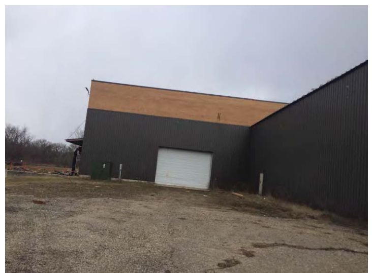
View north to a loading area on the west side of the newer warehouse portion of the mill.
