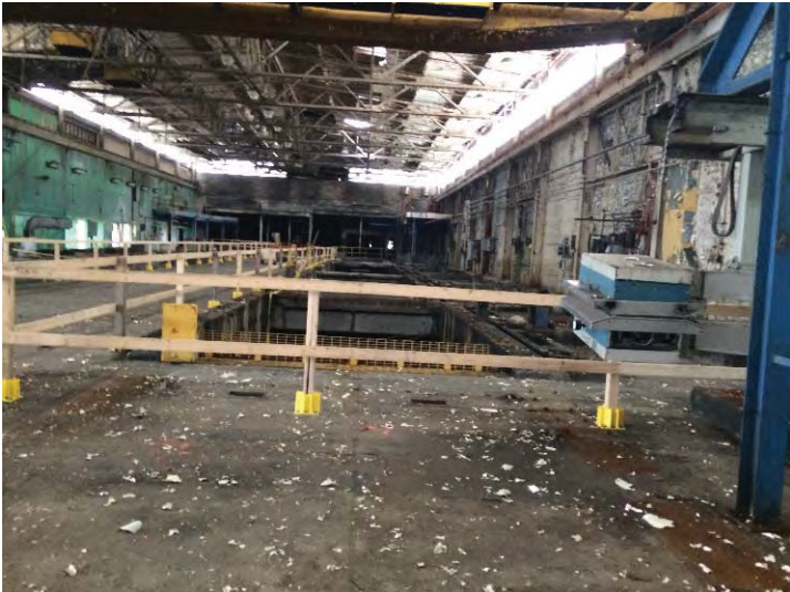
Former machine room in center section of the building.
