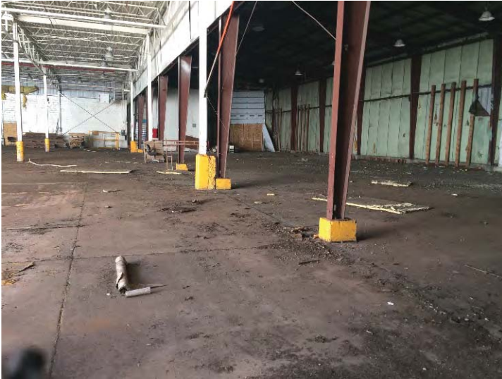
Newer warehouse portion of the building.
