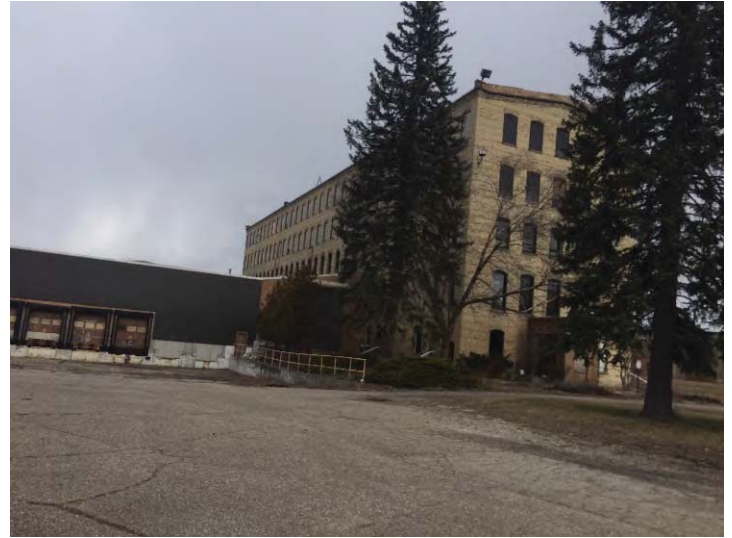
View north to the east wing and newer warehouse connection.
