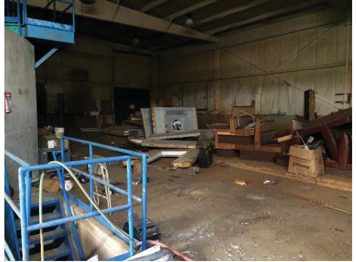
Interior of wastewater process building.
